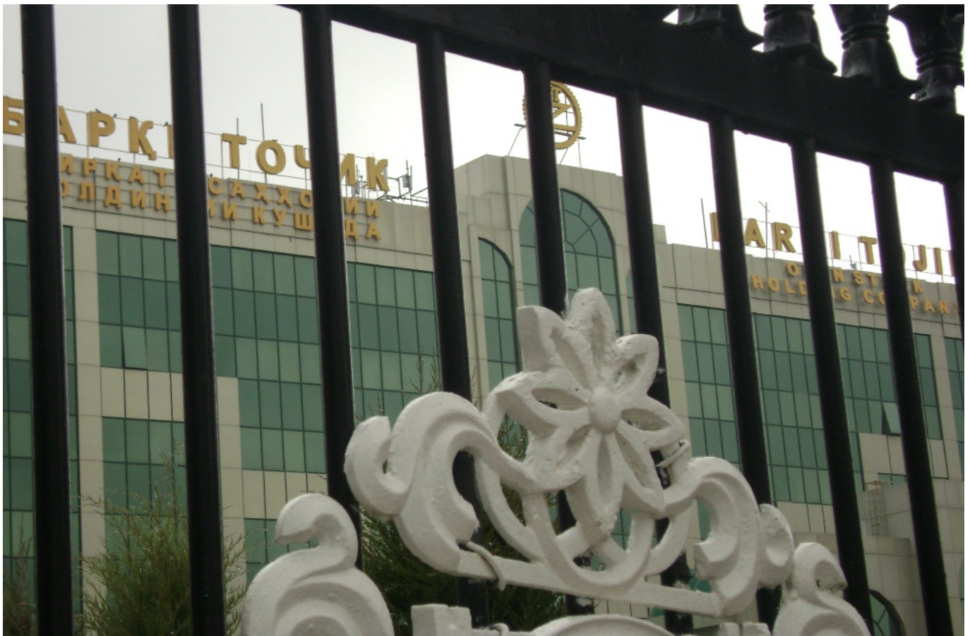
Administrative building of Barqi Tojik in Dushanbe, Photo: Asia-Plus
