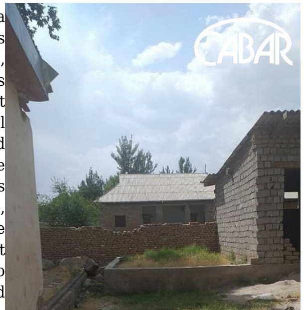
Today, the residents build their houses on the location of the former rural club in Jobi mahalla of the Oltinsoy district of Surxondaryo region. Photo: CABAR.asia
